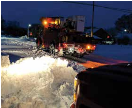
Crews worked into the night to ensure members power was restored.
