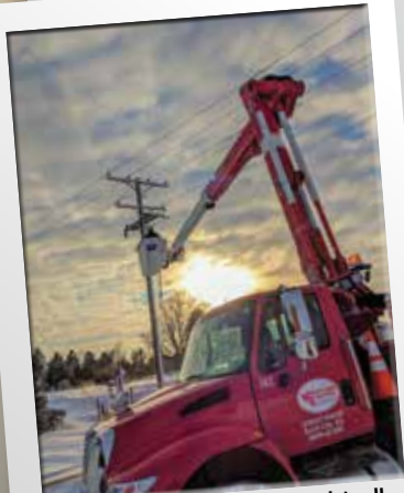
Wheatland Electric's linemen work in all weather conditions to get the power back on as safely and quickly as possible.
